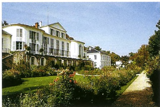
Figur 1. BIPM's hovedbygning, Pavillon de Breteuil. [1]
